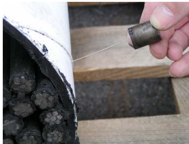
Fig. 2. Fuse wire connected to one of the strand inside the duct
