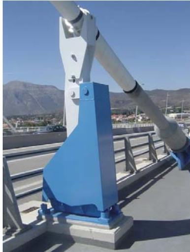
Fig. 6 Cable stays external hydraulic dampers
