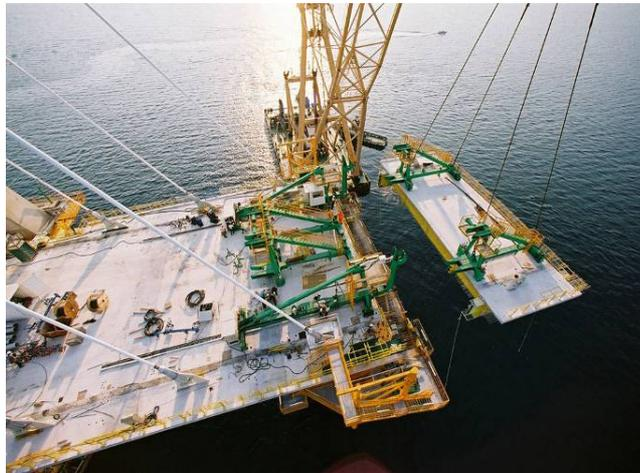
Fig. 6 Installation of a prefabricated deck segment
