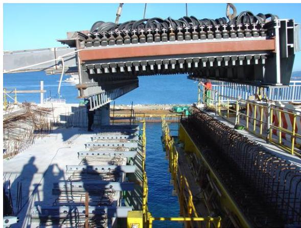
Fig. 10 Installation of MAURER expansion joint
