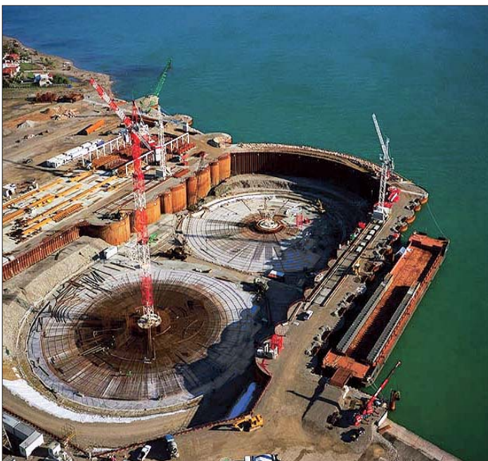
Fig. 12: Construction of pylonbases in dry dock
