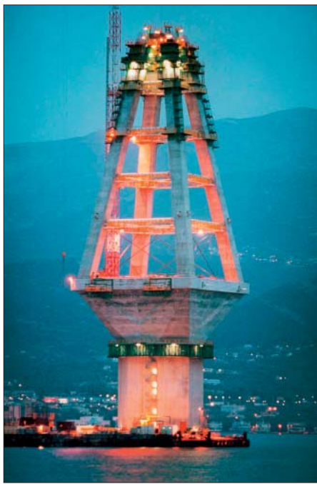
Fig. 14: Construction of pylon legs
